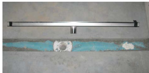
Linear Drain Install
